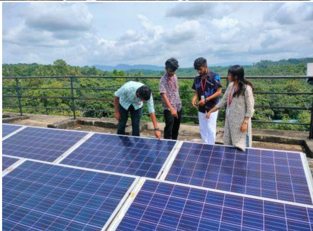
Solar Power Plant installed at the Administrative Block
